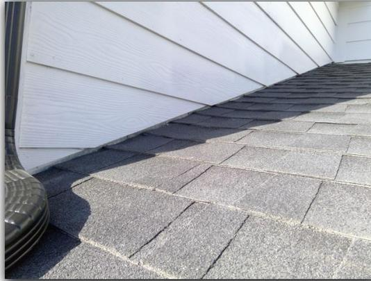
At the juncture of the roof and vertical surfaces, flashing and counterflashing shall be provided per the roofing manufacturer's Instructions. Provide a 2" clearance between the roofing and the bottom edge of the siding and trim.
